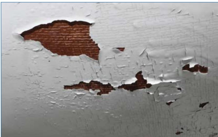
Poor preparation and painting caused this blistering.
